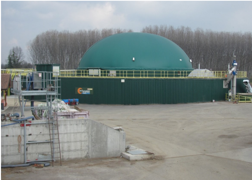
Figure 2. Anaerobic digestion system used in a swine farm in Northern Italy
