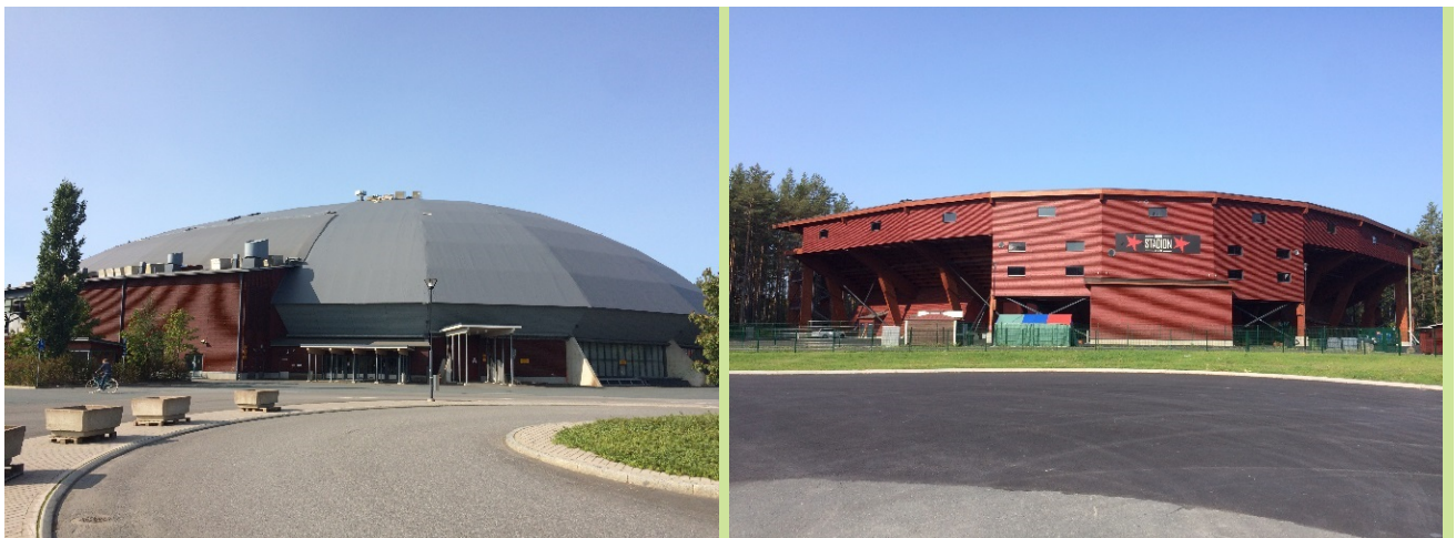
Wood in complex multi-functional public building: Sport Arena and Baseball stadium in Joensuu, Finland. Photo by Jan Kašpar
