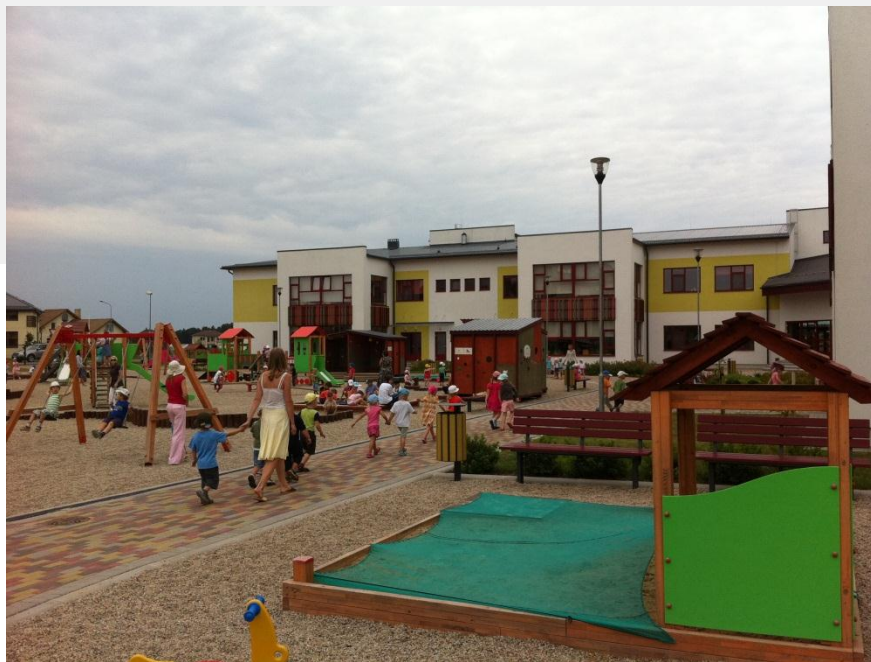
EUR 12 million Municipal Kindergartens (4) Project, Latvia
