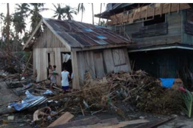
In the Philippines, cyclones and typhoons are so frequent that structural damage like this needs to be repaired before the next typhoon hits. © EC/ECHO/Bernard Jaspers Fajjer
