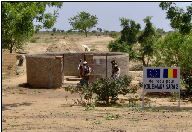
Waterhole construction in Kolemara Sara, Chad
