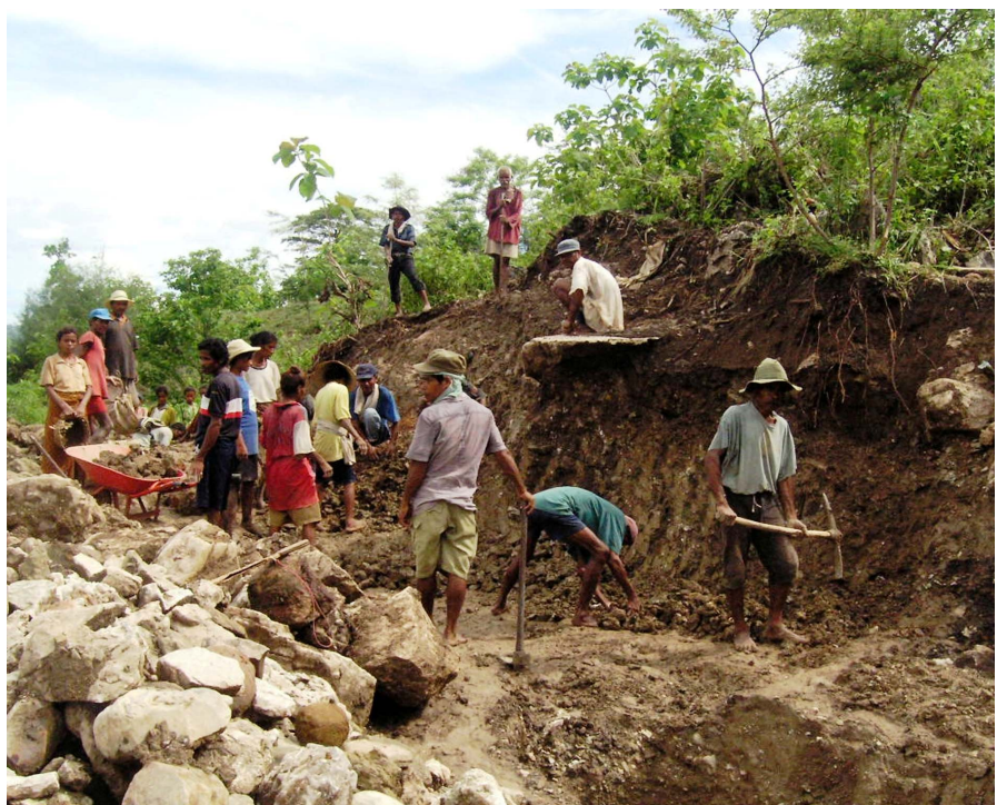
Rehabilitation of an eroded irrigation system, Lautem district
