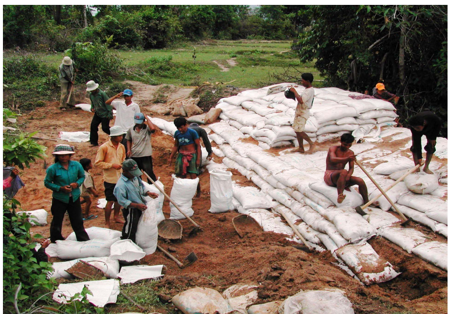
Community water control system under construction, Kampon Chhang
