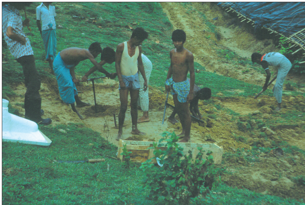
Drilling boreholes for latrines, Bangladesh
