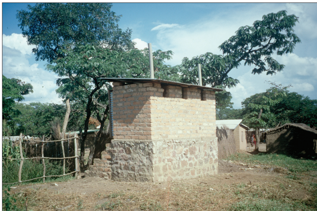
Raised VIP latrines, Tanzania
