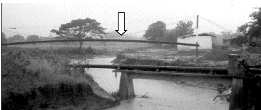
This photograph shows the effects of flooding during El Niño in Ecuador in 1999. The construction of a river overpass is a mitigation measure for piping.
