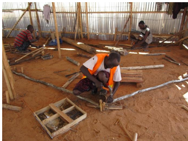
Picture 9: Construction of shelters
