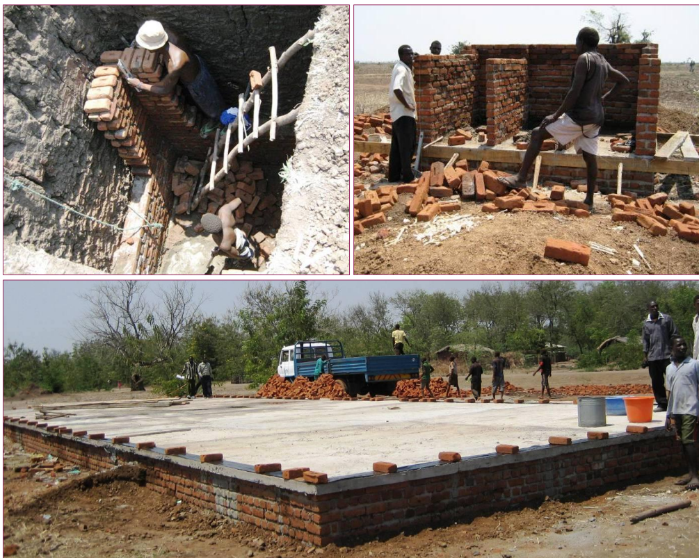
Figure 3 School or Evacuation Centre? Classrooms with kitchen and permanent deep latrines in Malawi
