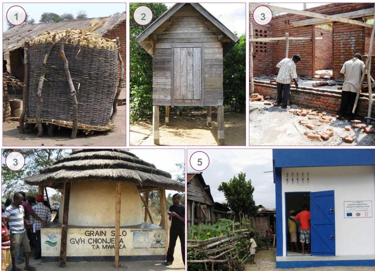
Figure 6 Different silo constructions: (1) Traditional unprotected silo (Malawi); (2) Silo with local material in Madagascar (relief funds); (3) Permanent Granary in Malawi (with office space); (4) Silo with local material in Malawi; (5) Concrete silo in Madagascar
