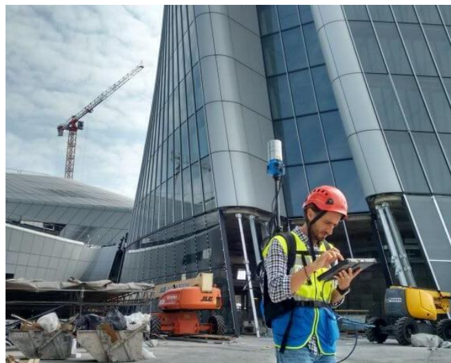
Figure 18: Italian start-up Gexcel 95 , in cooperation with the European JRC, has developed a backpack equipped with a 3D scanner for rapid mapping of indoor and outdoor sites
