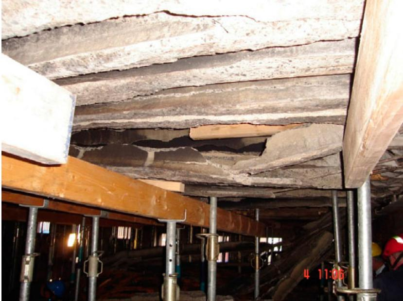
Fig. 5: Damage occurring in the car park fire at Lloydstraat Rotterdam (Fig. 25 from DE FEJTER/BREUNESSE [4])
