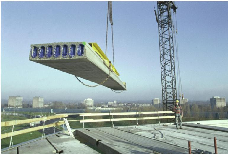
Figure 2: Example of prestressed concrete hollow slabs (CC BY-SA 3.0, SCHMAHL [5])
