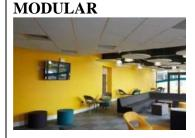
Modular ceilings are comprised of smaller tiles laid into a grid system from above and held up by the grid system without needing any permanent mechanical fixtures, therefore providing easy access to the technical equipment in the ceiling cavity by simply pushing up the tiles. These ceilings are almost exclusively installed in non-residential buildings.
