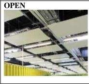
Open ceilings consist of a suspension and tiles, where the soffit and any technical equipment are only partially concealed by panels that are suspended within a grid system. These panels may have many different forms and shapes, such as canopies, baffles and clouds.
