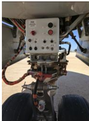
Figure 15: Landing gear maintenance box (source: Form CO)
