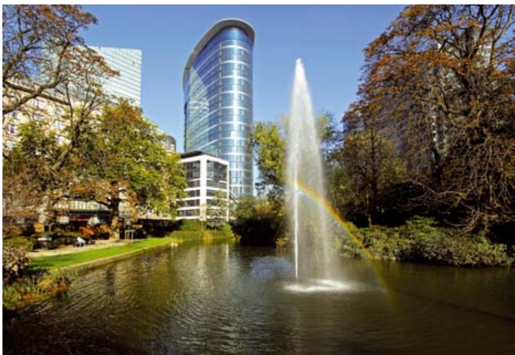
L'European Research Council (ERC). / S. BRISON, per cortesia d'Art& Build Architect / Montois Partners.
