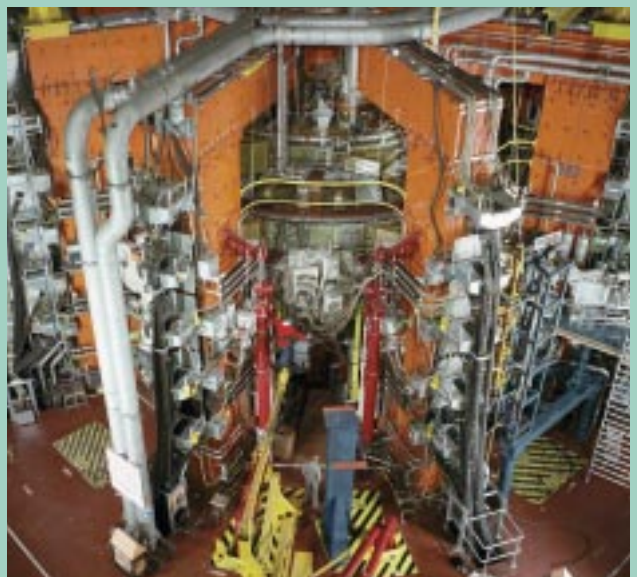
The JET plant during the transformation operations
