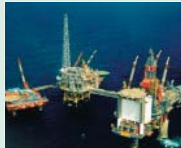
Sleipner West natural gas field where separated CO 2 is being injected into a deep salt-water reservoir (Courtesy of Statoil).
