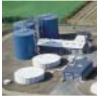
Ribe Biogas plant in DK (Krüger©).
