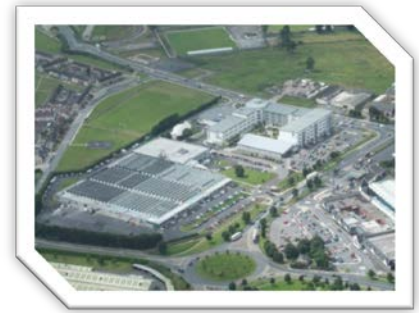
LEDP's 16 Acre Facility at Roxboro
