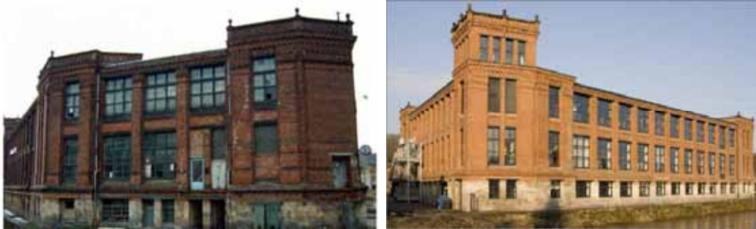
Figure 2: The Wasserbau (before [left] and after [right] the reconstruction)
