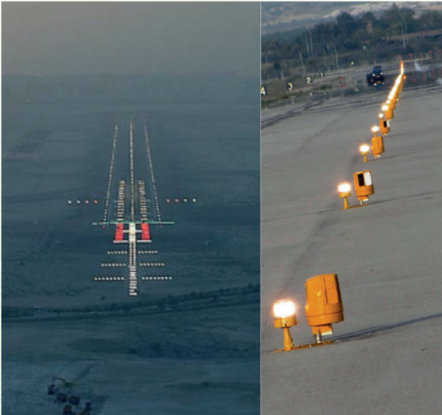
Airfield Lighting Installations
