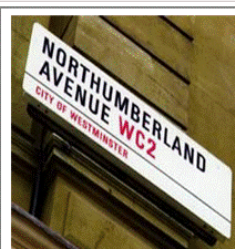
Street sign encloses microcell antenna
