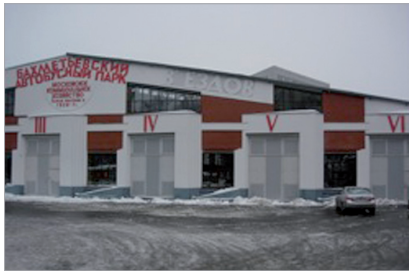
Bakhmetevsky Bus Garage, 1927. Architect Konstantin Melnikov, engineer Vladimir Shukhov
