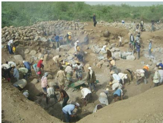
Building a water harvesting system, Al Hodeida Governorate
