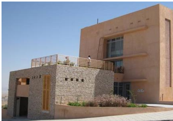
An energy efficient building designed for hot dry climate in Aqaba, Jordan. This MED-ENEC pilot project is the national winner of the Energy Globe Award 2007.
