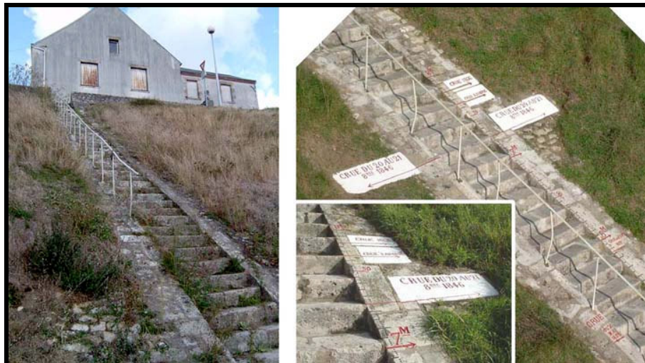
Flood scale in the Loire basin (F), before and after restoration
