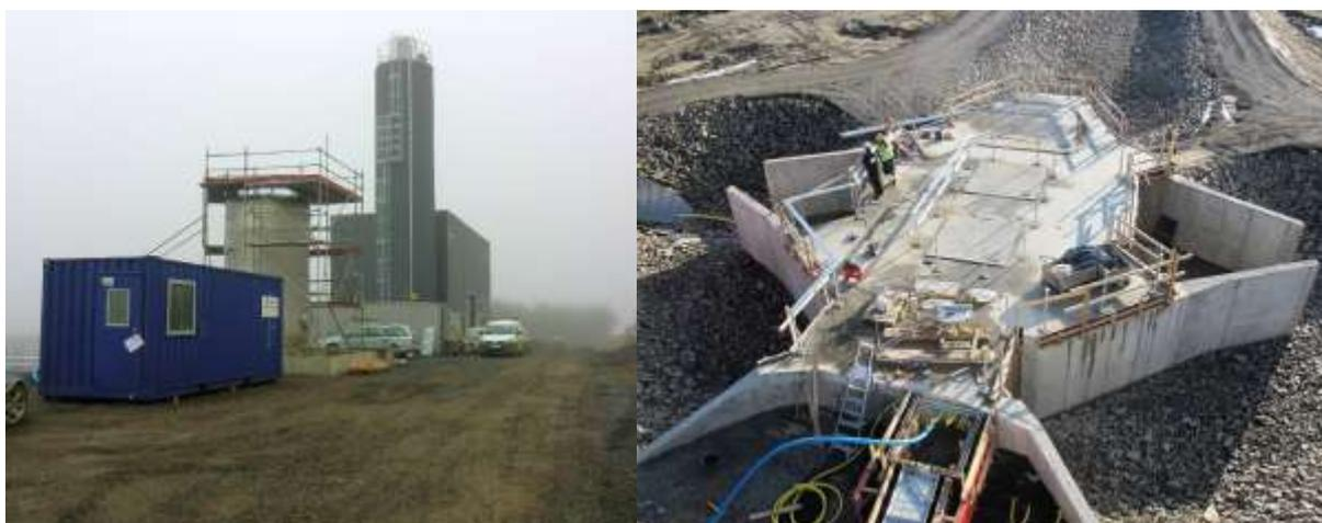
Figure 2 Treatment facility under construction for treating thiosalts using the Fenton-process at the Hötjäm TMF in northern Sweden.
