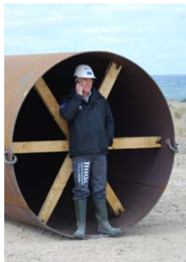
Test pipe before installation
