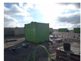
On-line control of the recirculation system
