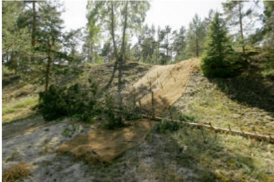
*Figure 6. Fixing eroded soil*
