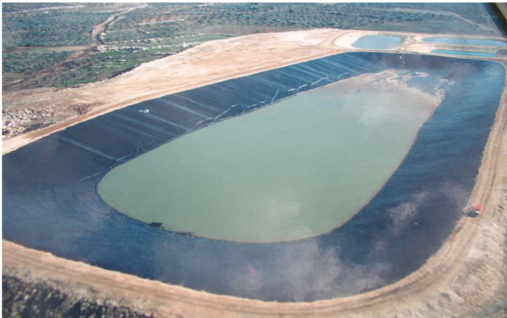
Figure 1. Available wastewater treatment plant of Sakhnin.
