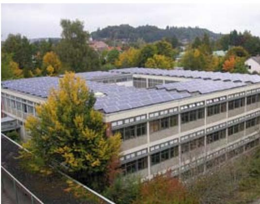
The roof of the Leutkirch school is covered with photovoltaic panels. The electricity produced is dispatched to the city net.
