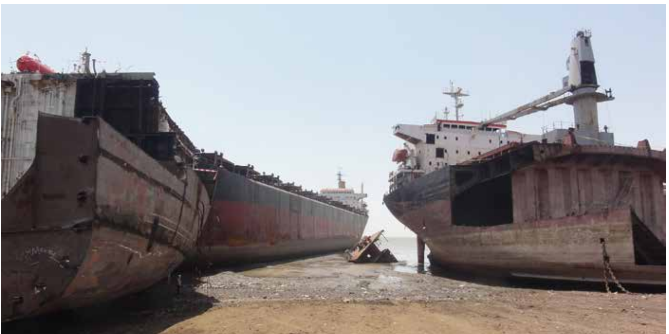
Ship being broken, Alang, Gujarat, India.
