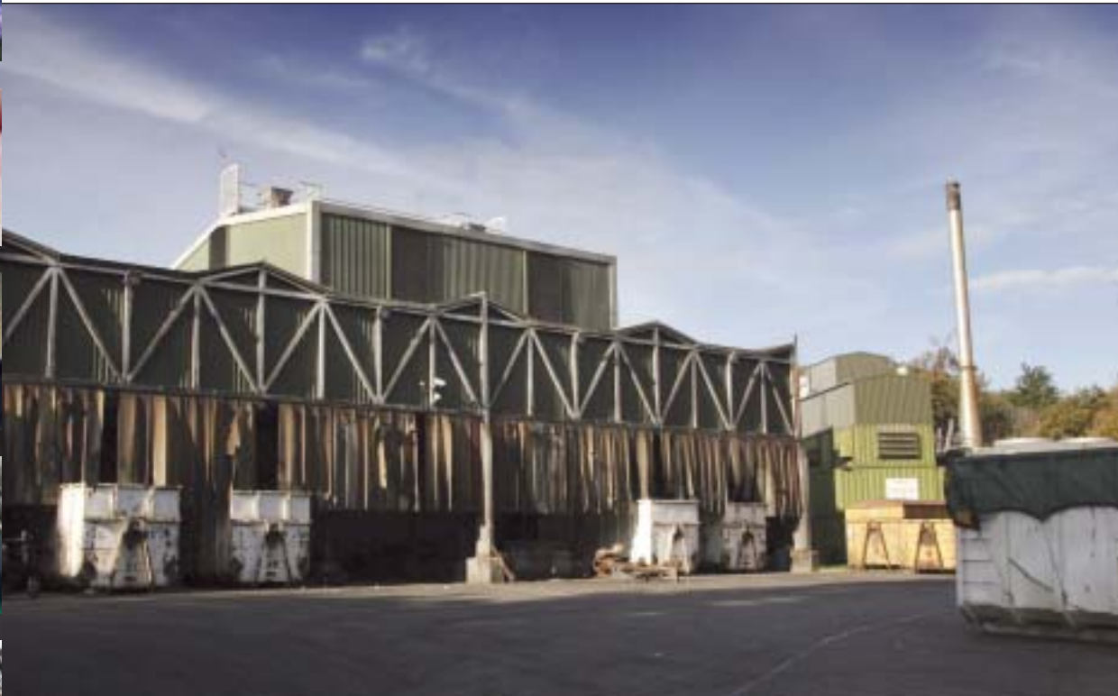
The Resource Recovery Facility.
