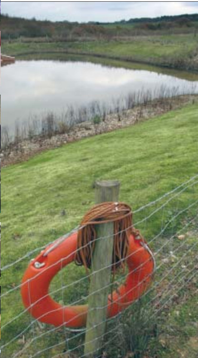
Attenuation pond at Standen Heath landfill site. Patrick Eden
