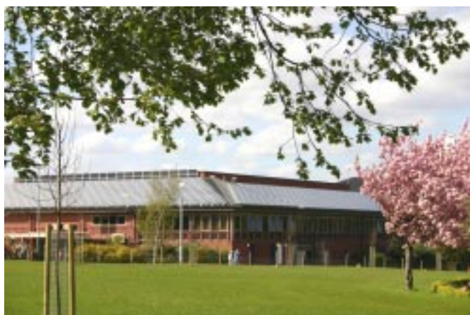
Solar panels on Queen's Park Sports Centre
