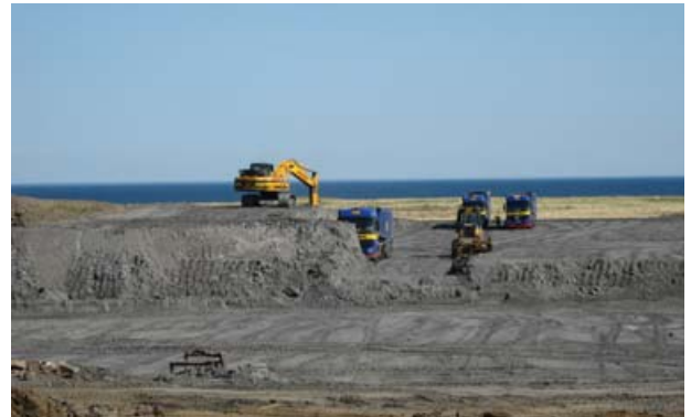
Articulated lorries waiting to be loaded with ash.
