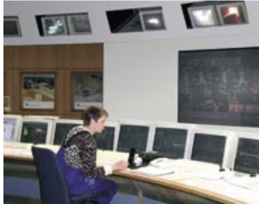
Inside the central control room
