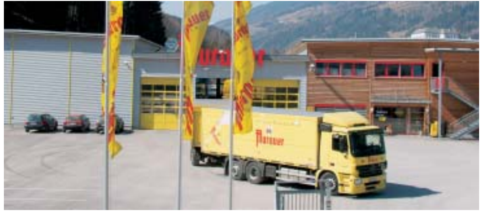
Environmentally friendly: the Logistics Centre was constructed according to ecological principles
