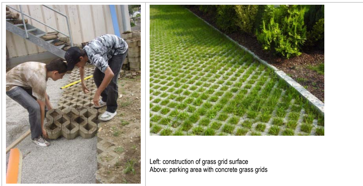
Fig. 70 Concrete grass grids – examples
