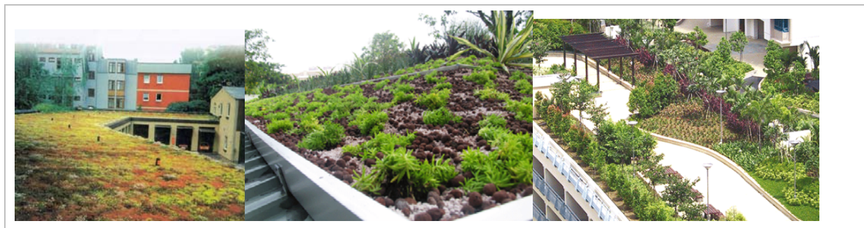
Fig. 76 Green roof types: extensive, semi-intensive, or intensive
