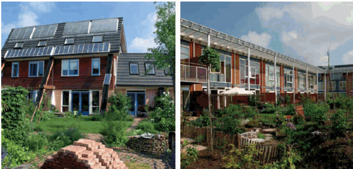
Fig. 50 Innovative housing: examples of private housing initiatives. Left: Semi detached houses with sun panels for photovoltaic and heating. Right: Row houses with joint landscaping. Source: VROM [77]
