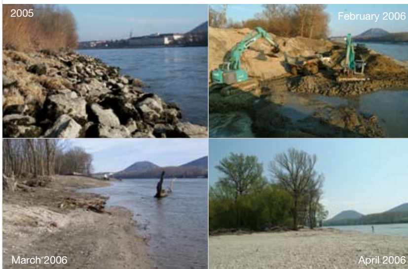
Original site (top left), stone embankment removal (top right), after the machinery (bottom left), and the effects of erosion (bottom right)
