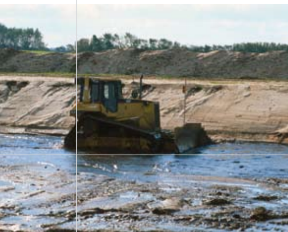
Reconstruction work on the River Skjern
