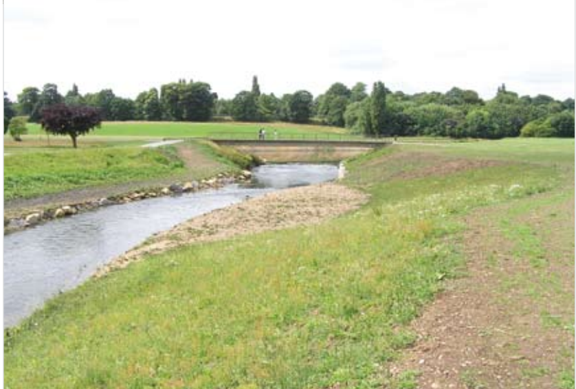
The banks of the river were lowered to allow the river to follow a more natural course
