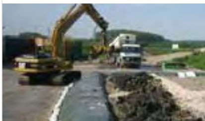
Deposition of extracted sediments following TBT removal
