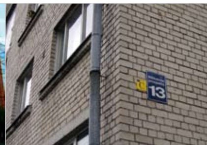
Clearly visible energy labels (from A to E) indicated the buildings' energy consumption.
