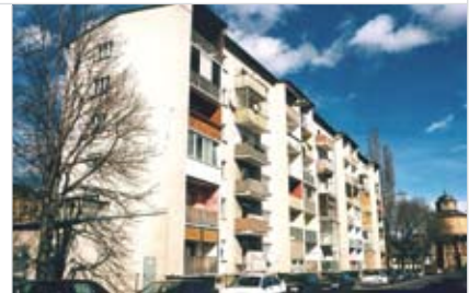
The Daungasse estate before award-winning retrofitting and renovation.
