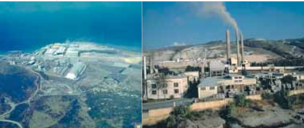
Cement works in Lebanon.
