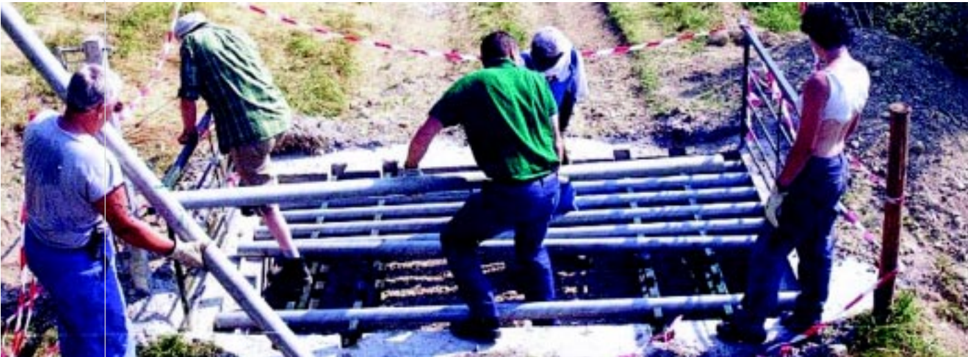
Installing cattle stops on the Plateau de Millevaches. Photo © CEPA
