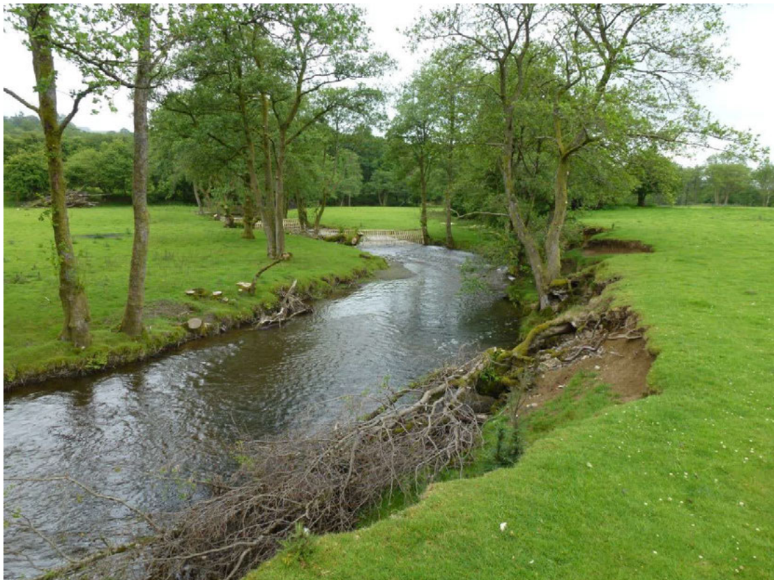
Figure 11; © John Houston : Riparian Bank Works on Farmland on the River Irfon
