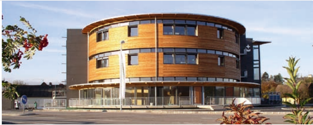
The Christophorus House's prominent circular form results in a compact building, with a reduced surface area and, therefore, lower energy loss.
