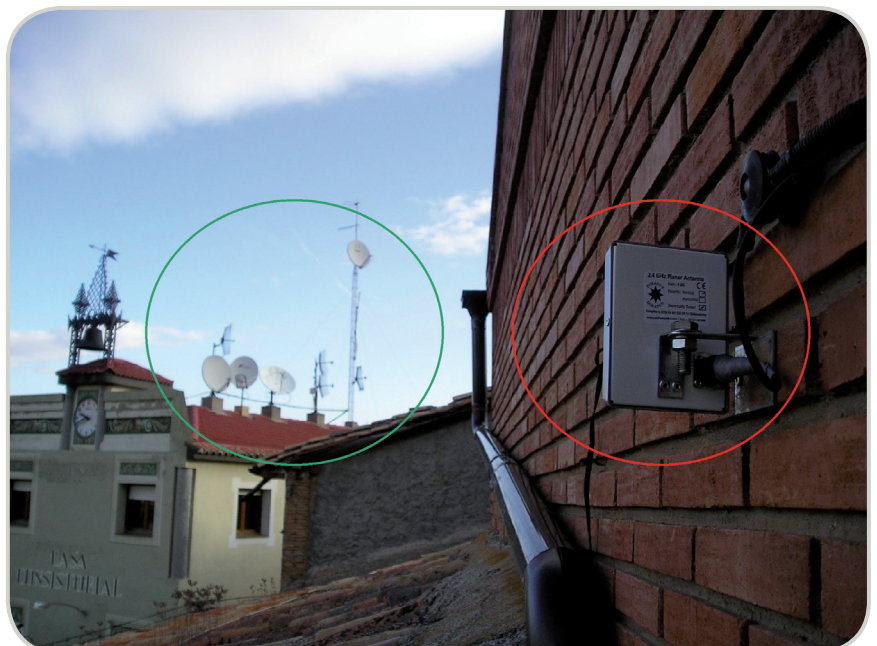
Satellite backhauling and central wireless base station Source: TWISTER
