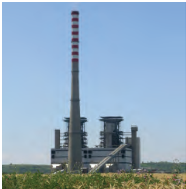
Kostolac B power station
