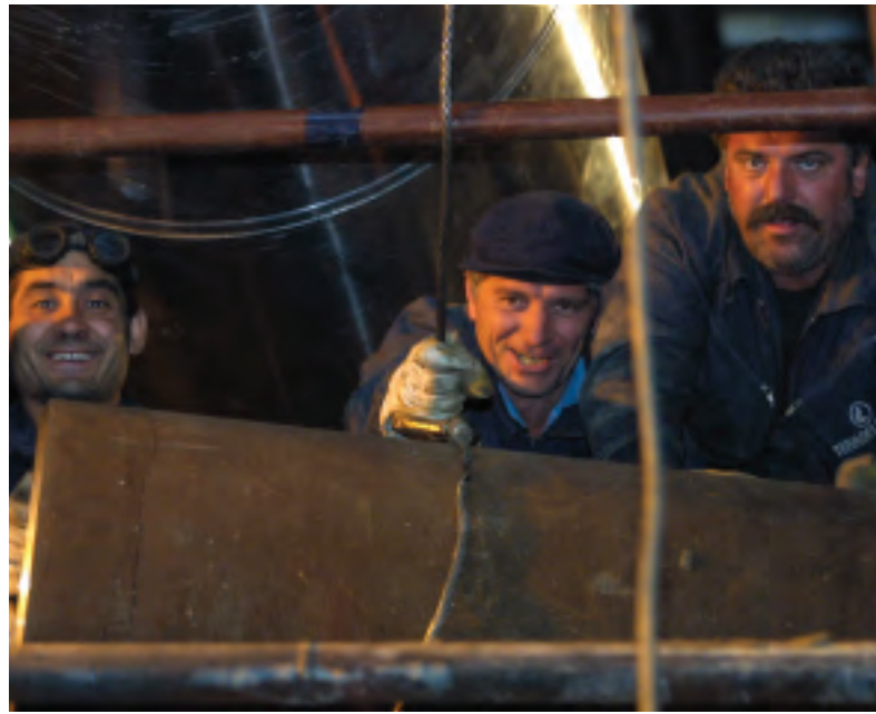
EPS workers installing equipment
