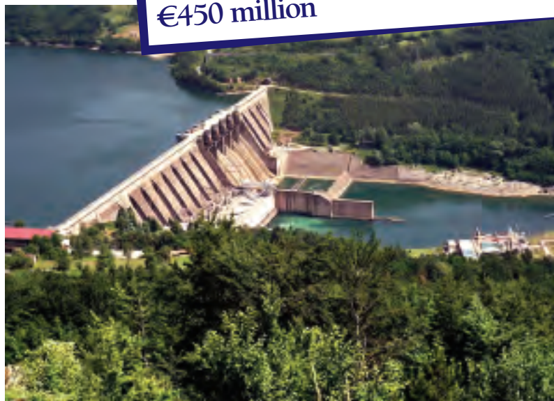
Bajina Basta hydro-electric power station
