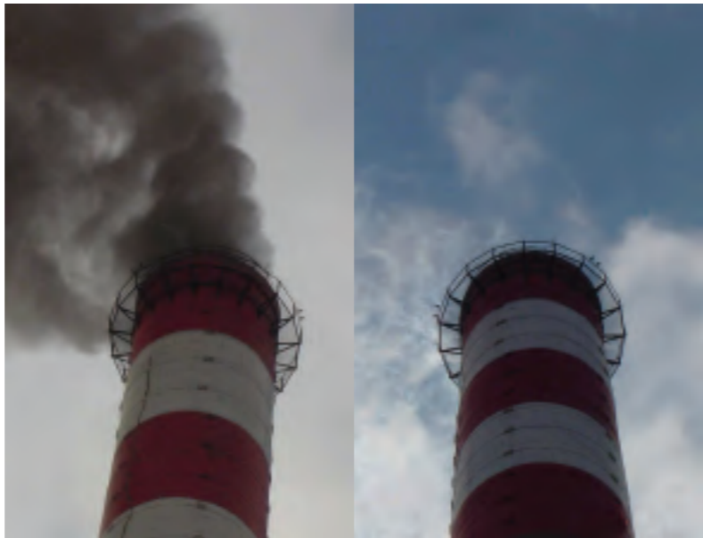
The main chimney of part of the Kostolac power plant in eastern Serbia before and after installation of electrostatic filters. The filters, installed at a cost of €5 million as part of the Agency's energy programme, will reduce emission of dust and other pollutants to below the EU minimum standard. This will result in cleaner air for a region of 100,000 people.
