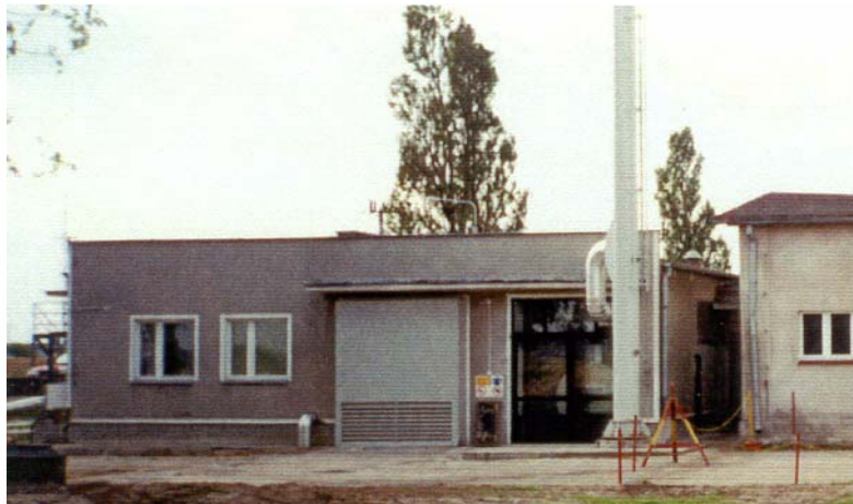
Photo 1: The Combined Heat and Power plant
