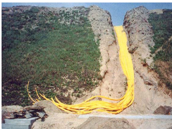
Photo 2: The gas extraction lines and their connection to the pumping module during the construction phase
