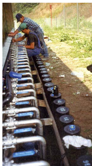
Photo 2: The gas extraction lines and their connection to the pumping module during the construction phase
